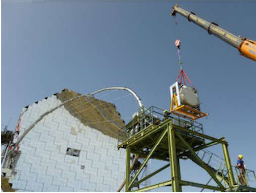
Fig. 7: Installation of the new MAGIC-I camera
